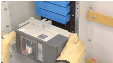
The Breaker Is Inserted Into The SafePanel
