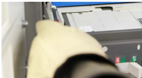
Screws Help Secure The Breaker
